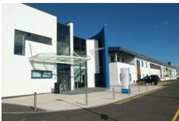
Crosshouse Maternity Hospital, UK
